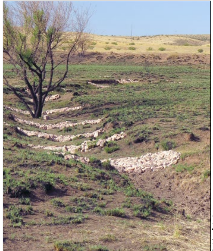
Low-profile erosion control structures retain soil and moisture.
